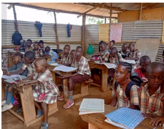
Temporary corrugated iron classroom
