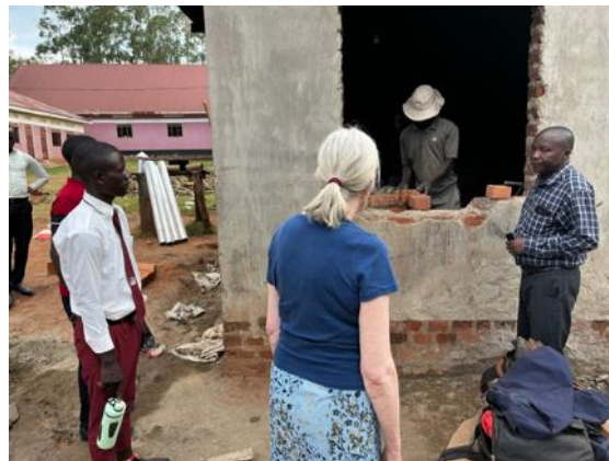
Mustard Seed kitchen during construction in 2024
