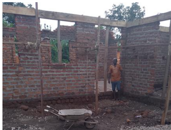
Construction of girls' dormitory
