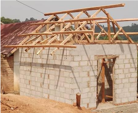
Work on new Lily van Haelen toilets
