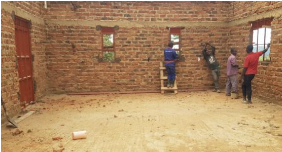
Work on Kanungu School Hall
