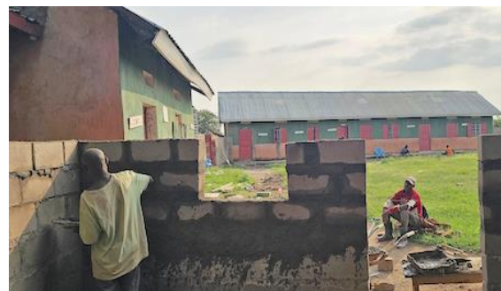
Refurbishment work at Kahendero school
