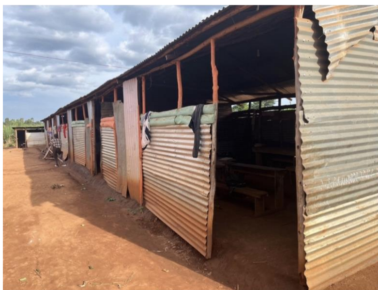
Corrugated iron classrooms at Eagle's View School
