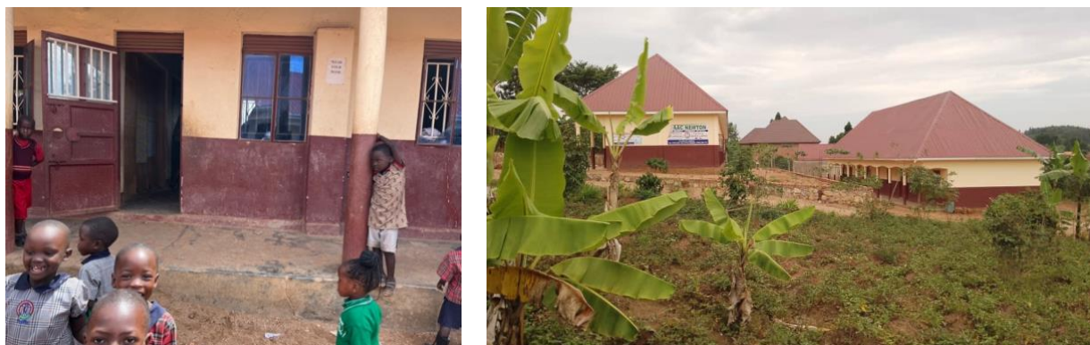
Old site with unsafe buildings (left) New site with fine new classrooms (right)
