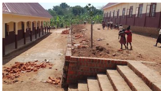
Soil stabilisation & drainage work between the new Junior and Infant Annexes
