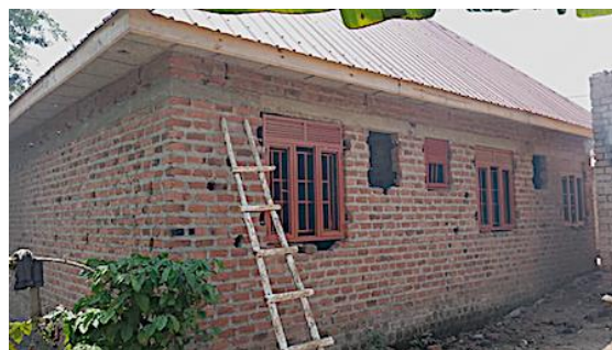
Finishing work on the Teachers' House – a community initiative
