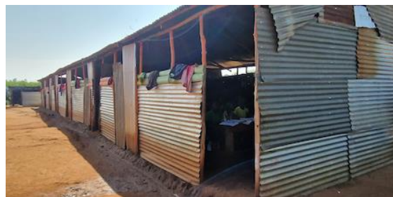
Cookhouse and temporary classrooms
