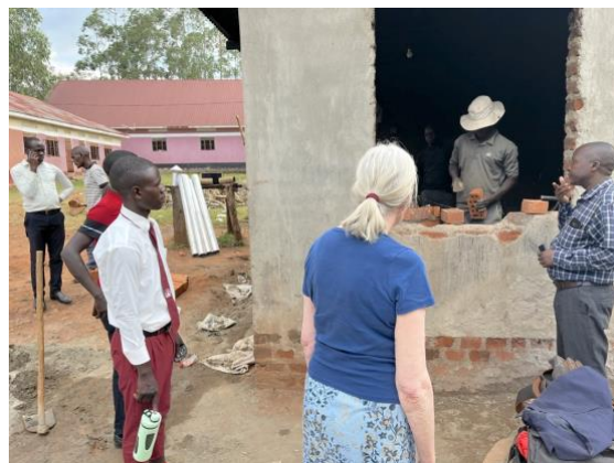
New kitchen construction
