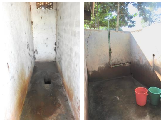
Boys' pit latrine & shower room
