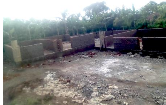
Outside walls of 3 Nursery Classrooms
