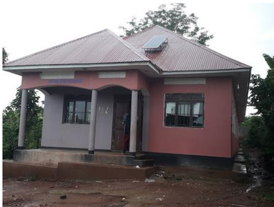
Entrance to new girls' dormitory
