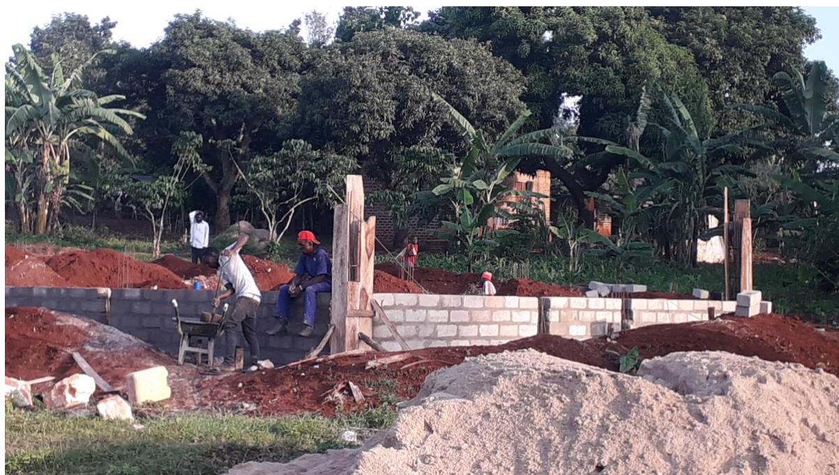
Foundation work on new Boys' Dormitory
