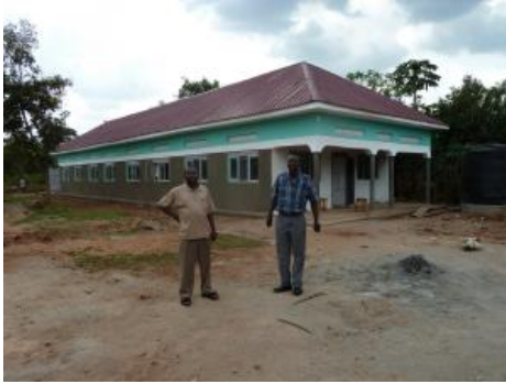
Girls' dormitory nearing completion
