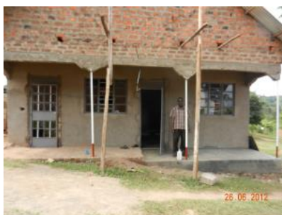
Teachers' dormitories under construction (the new kitchen is behind)
