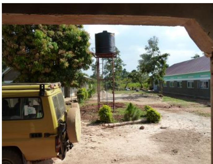
Pumped water system and girls' hostel at Mustard Seed School
