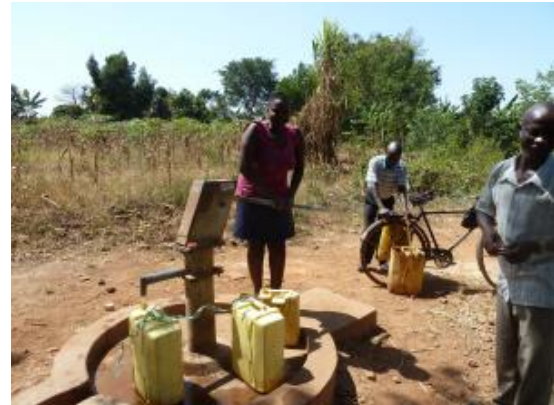
New borehole providing fresh water to Mustard Seeds upper school site
