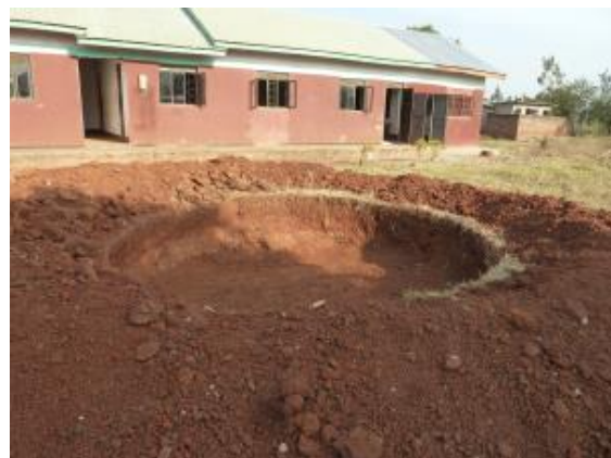
Hole being dug at Mustard Seed for underground concrete water tank
