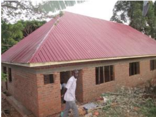
Isaac Newton Boys' Hostel under construction
