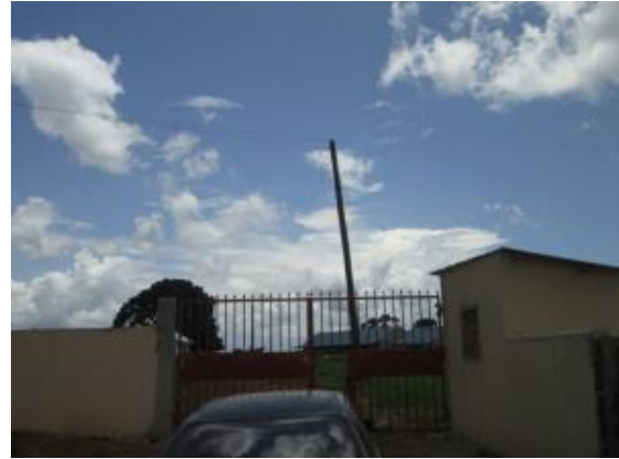
New secure gated entrance to Mbute Campus
