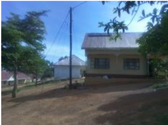
Power cables to the computer lab
